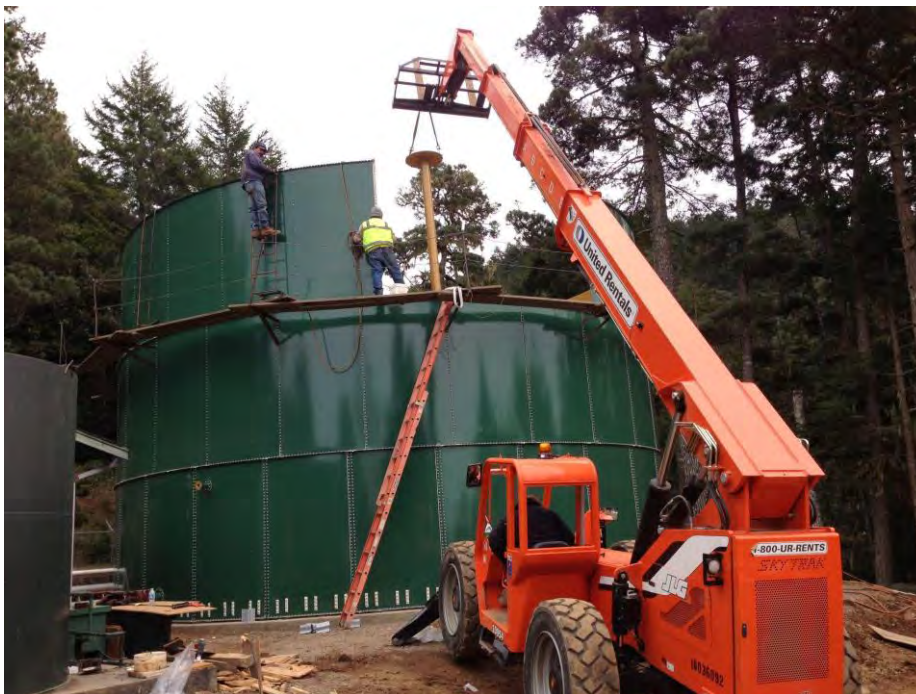
Tank under construction
